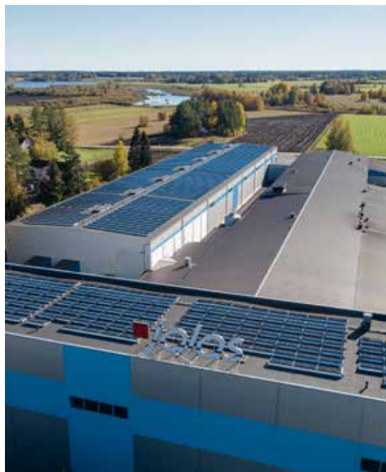
During 2021, we installed a 400+ MWh/year solar panel system in Jokipii, projected to give 20% of the site's annual electricity need.
